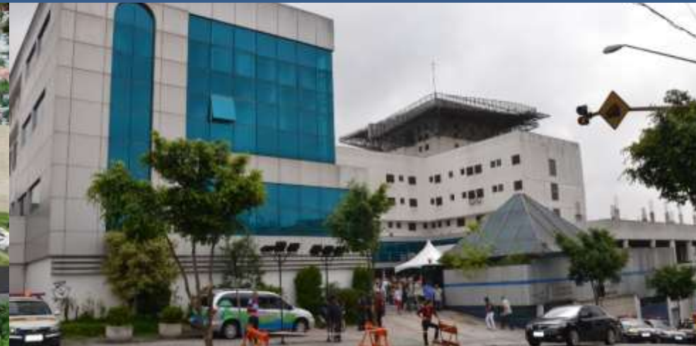
Hospital Municipal Vila Santa Catarina
